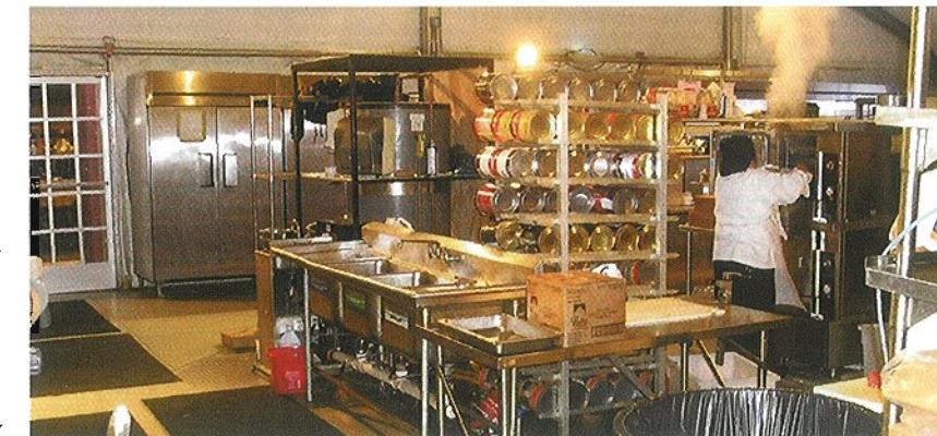
To support the bulk cooking, the production kitchen is equipped with two roll-in combi-steamer-ovens, six rack combi-steamer-ovens and pressure fryers.
